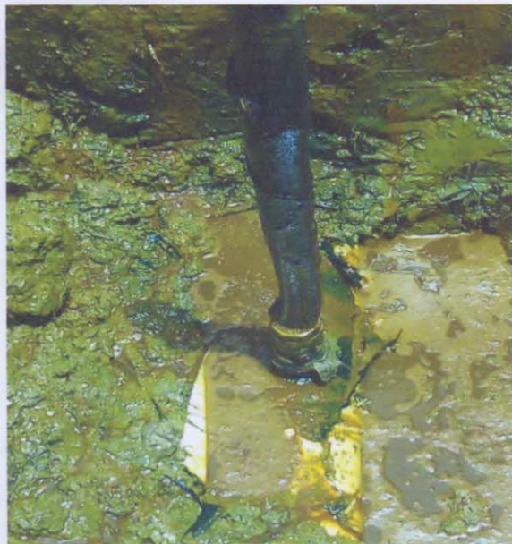
Figure 2: AFTER EXCAVATION 2" VALVE FOUND
